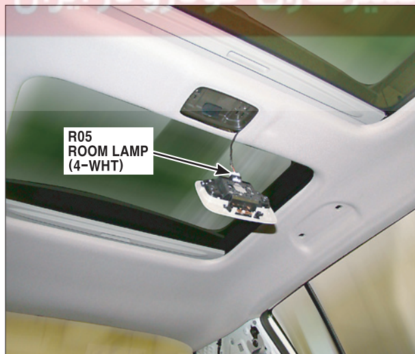
100. Center of Roof Trim
